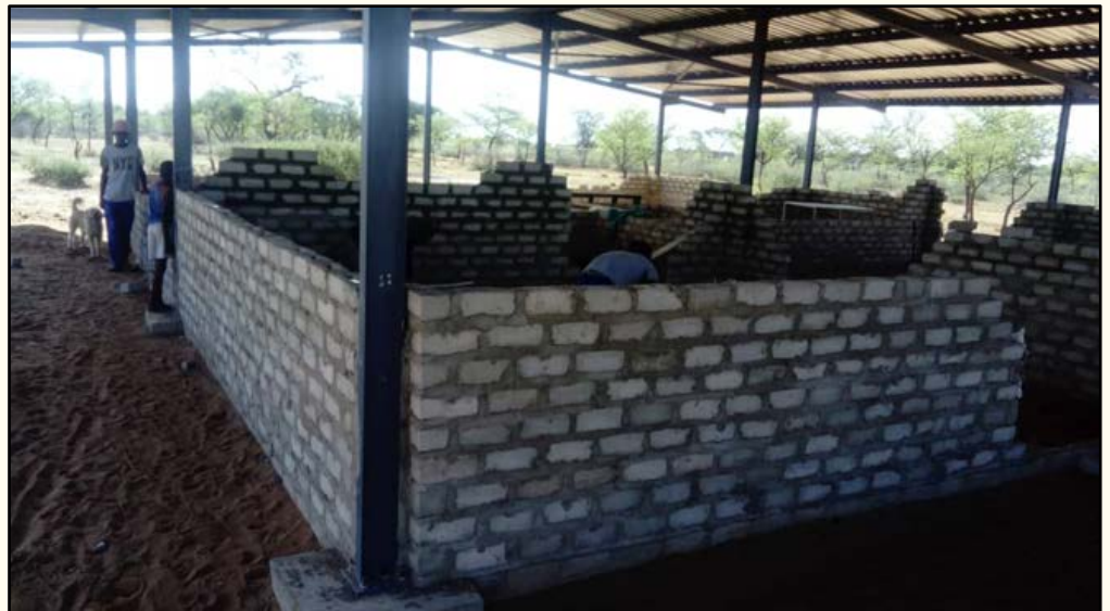
Resource Center Construction – supplied by Helge Mercker
